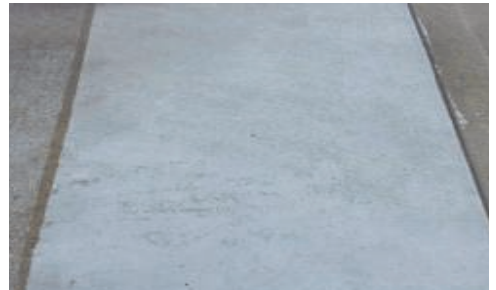
FIGURE 7—New acrylic latex garage floor coating applied to concrete pad after five months (cleaned).
