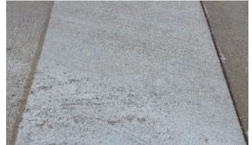
FIGURE 6—New acrylic latex garage floor coating applied to concrete pad after five months (uncleaned).
