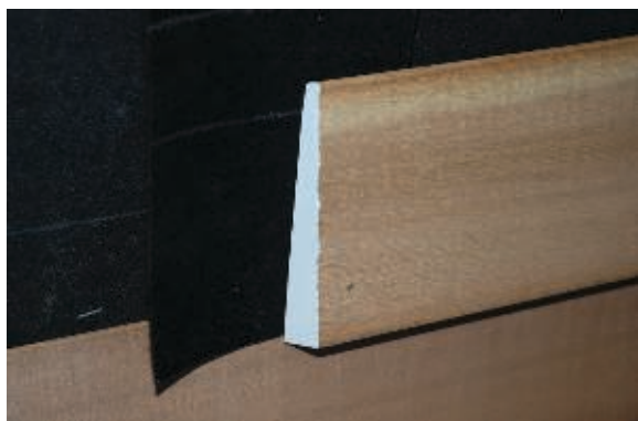
Figure 5—A 45° bevel joint on rain screen construction showing a primer applied to the end grain and interleaved water-resistive barrier.
