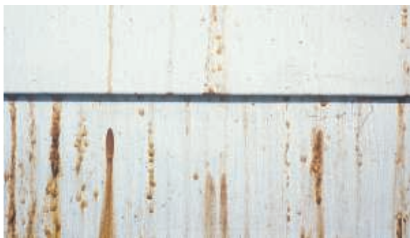
Figure 2—Extractive bleed of siding caused by wetting the back side of unprimed siding.
