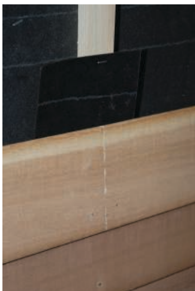
Figure 6—Completed joint. Note that fasteners are approximately one inch (25 mm) from the bottom edge of the siding and spaced well away from the end of each board. Nails were angled slightly to penetrate the furring strip and the underlying sheathing and wall stud.
