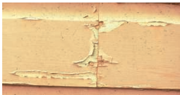
Figure 3—Water absorption into the end grain of siding caused the finish to peel. Note also that fasteners are too close to the end of the siding.
