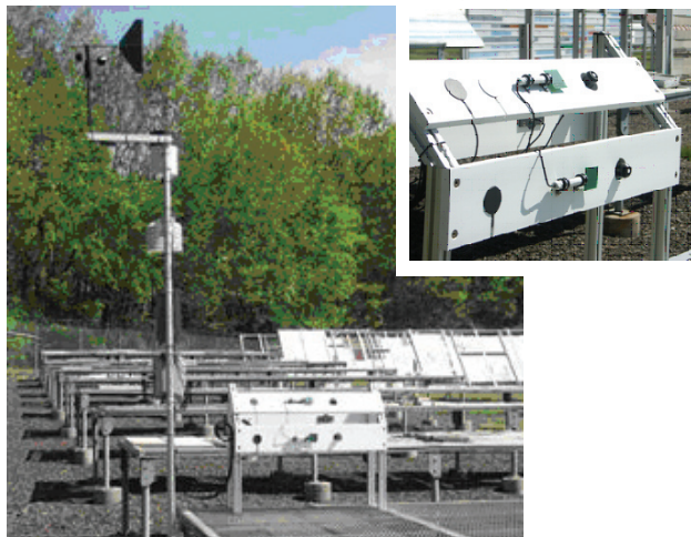
Figure 1—Weather station and directionally dependent sensors.
