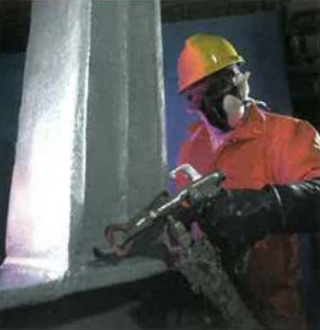
Fabrication shop application of Interchar fireproofing material to structural steel beams. Photo courtesy of International Paint Protective Coatings.
