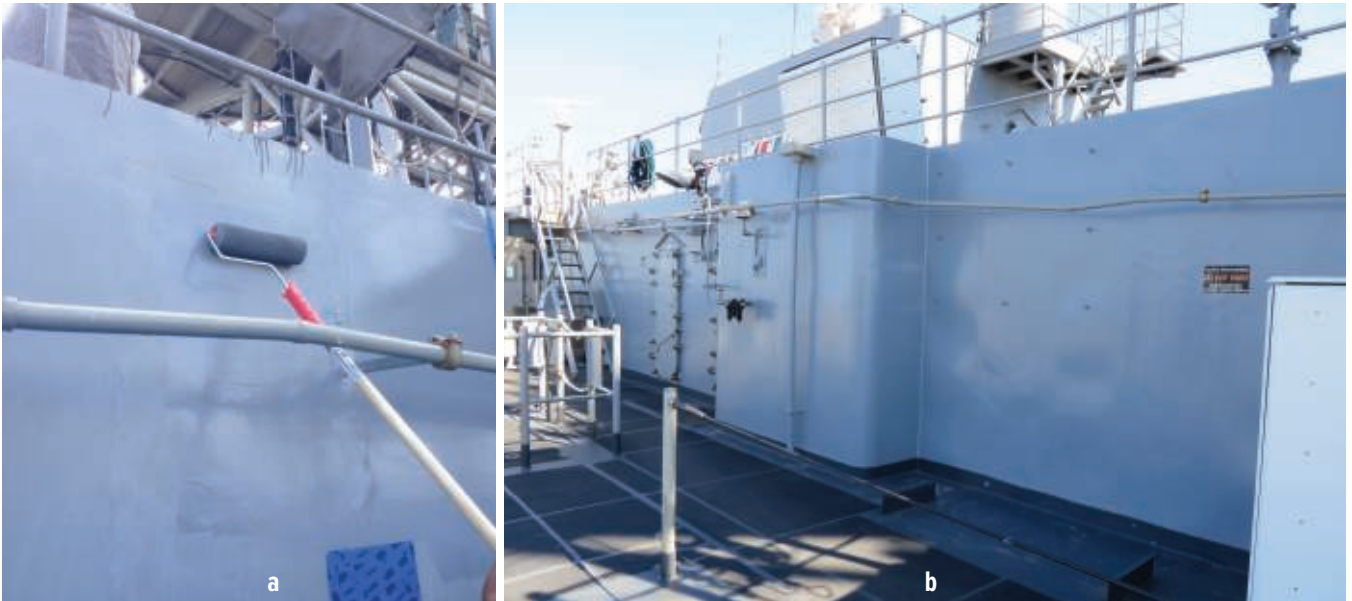
FIGURE 6—NRL's 1K polysiloxane topside coating on the USS GUNSTON HALL (LSD-44); a: roll-application over abraded silicone alkyd, and b: after six months of service.
