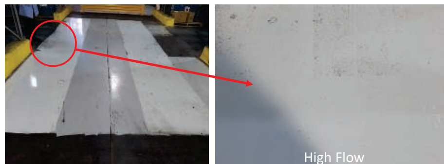
FIGURE 15—FCT applied to warehouse floors.
