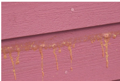
Figure 11—Large pitch pocket or seam.
