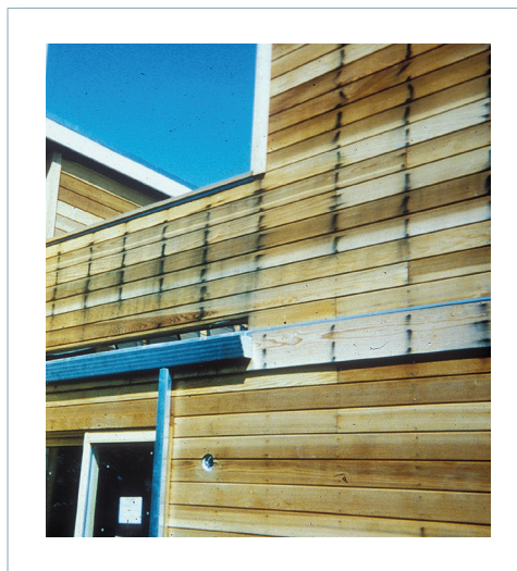
Figure 7 —Iron stain around electro-plate galvanized fasteners.
