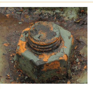
Figure 2 —Bolt and nut assembly on an Endicott gun emplacement containing lead.
