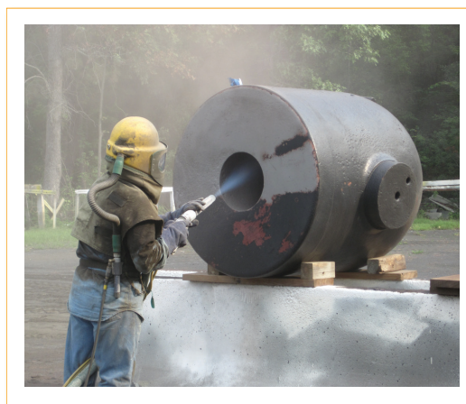
Figure 3 —Abrasive blasting performed on mortar tube by Phillips Industrial Services.
